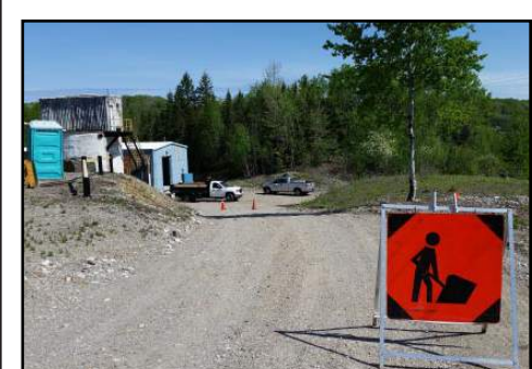
Construction at sites: Site closed
